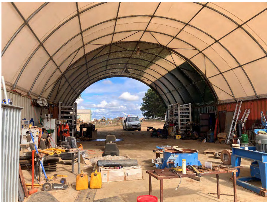
Photo 14: Maintenance workshop, looking south.
