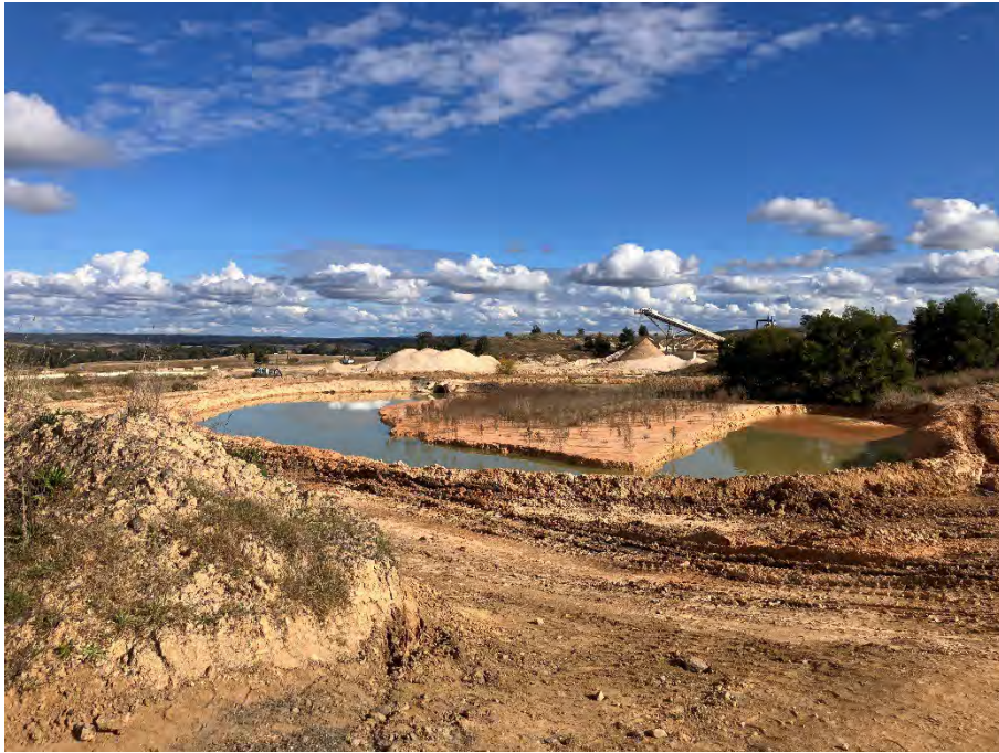
Photo 5: Sand processing plant and product storage, looking southeast across the upper Reuse Pond.
