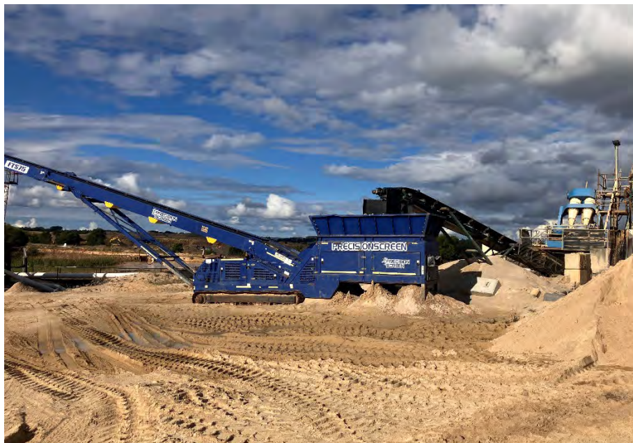
Photo 6: Sand processing plant and product storage, looking south.
