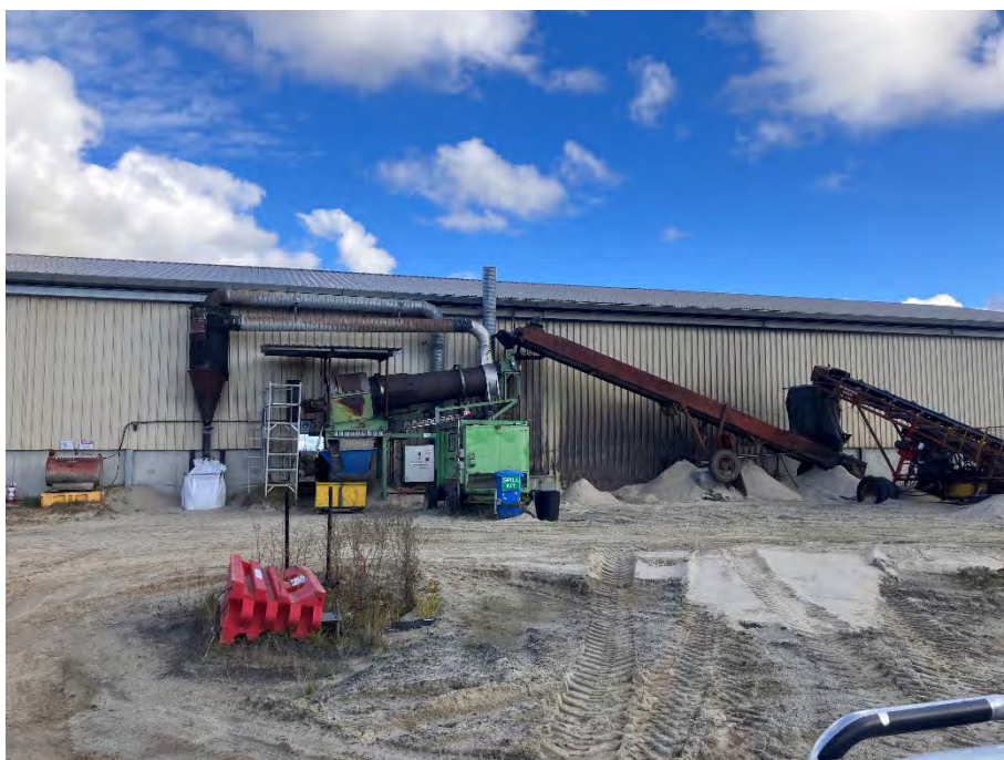
Photo 16: Sand drier and storage shed, looking south.
