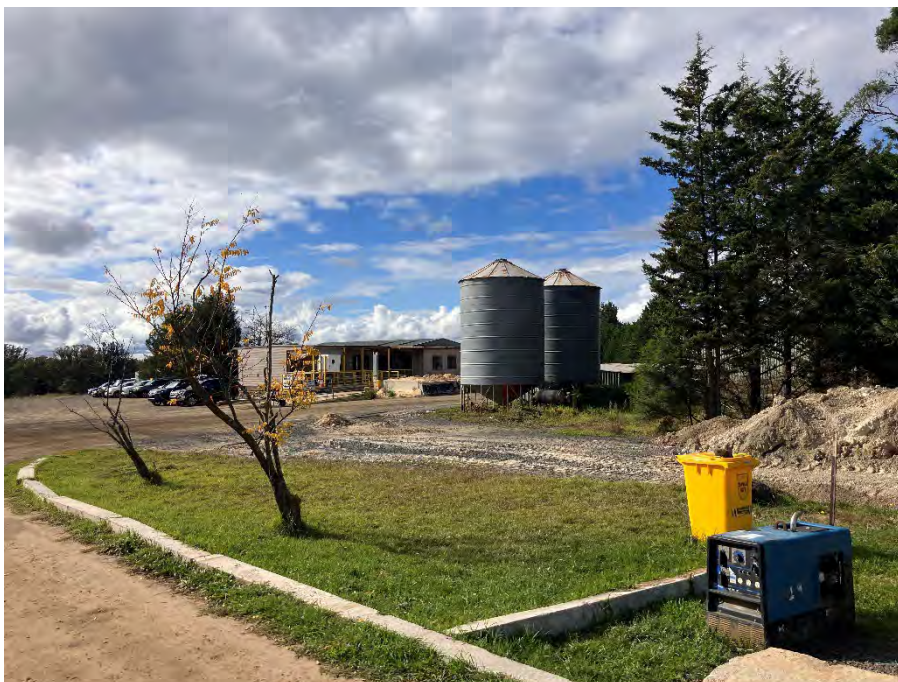
Photo 2: Office and weighbridge buildings, looking northeast.
