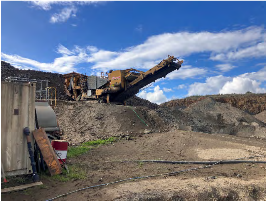
Photo 11: Basalt processing equipment within Basalt Extraction area, looking northwest.
